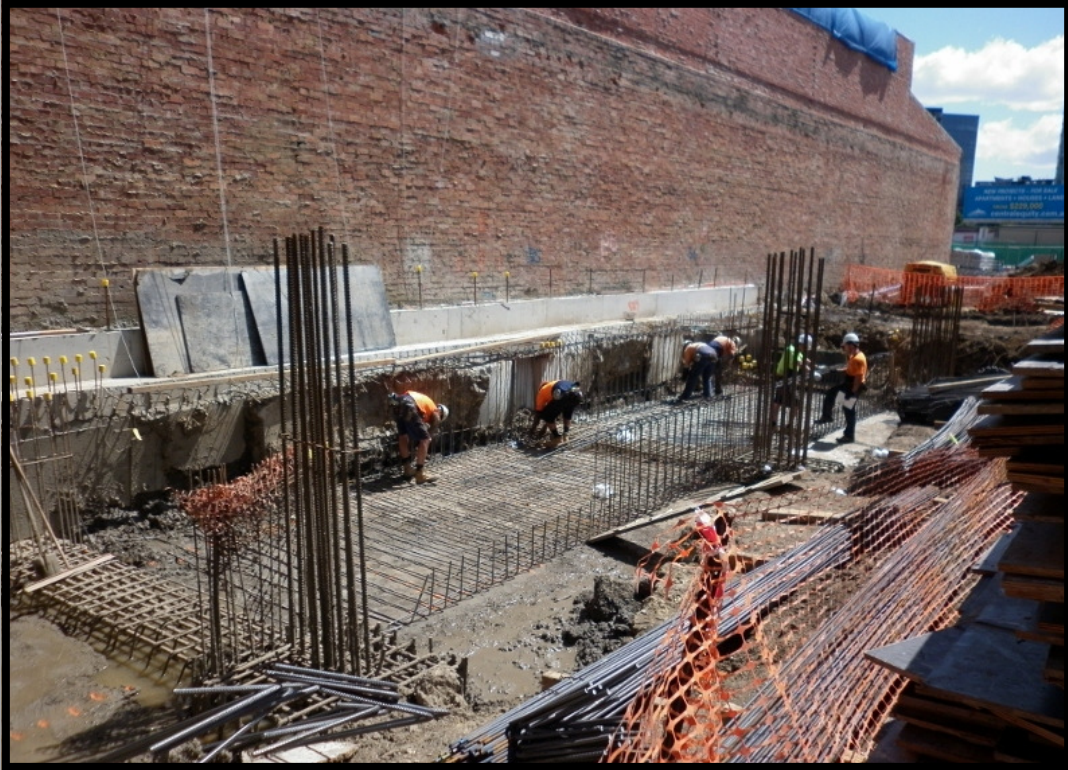
Construction on Guild's swimming pool
