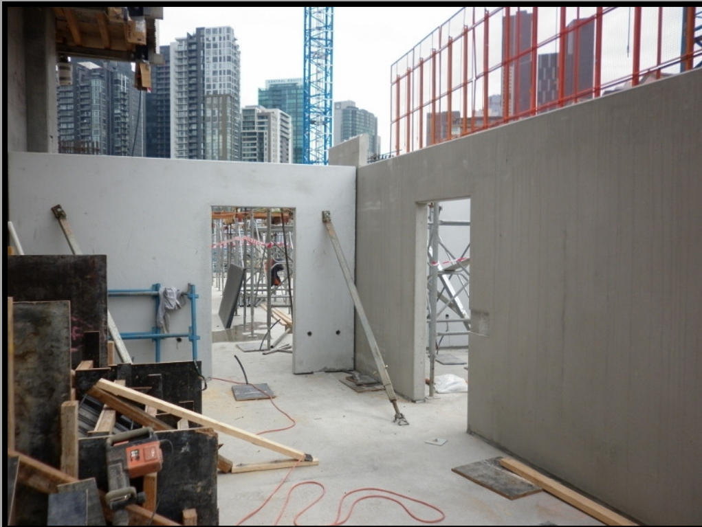
First internal walls on Level 1
