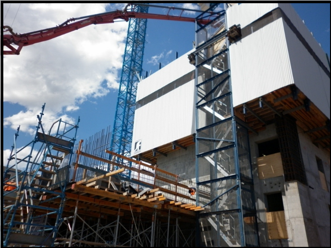
West tower core
