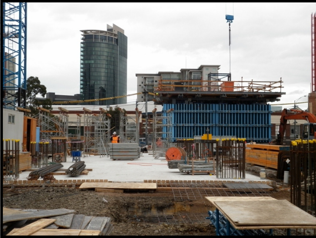
East core jump—prior to Level 1 being laid
